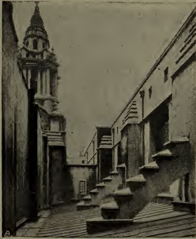
FLYING-BUTTRESSES AND SCREEN-WALL.
